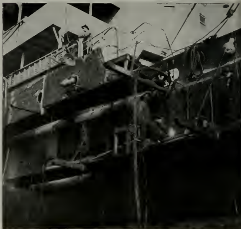
Sheerstrake doubling plates being butt welded.
